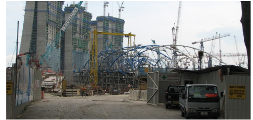
Recent shot of bridge in front of MBSIR.
